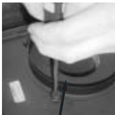
REMOVE FLUE RING
